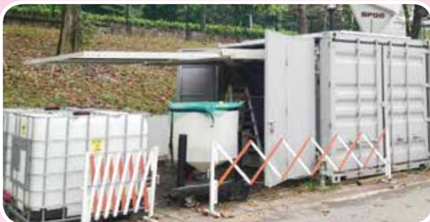
Solar-powered water generator (ultra-filtration).
