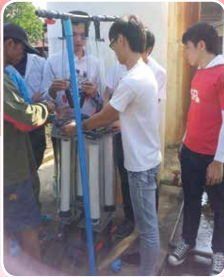
Students working together with villagers to install water filters.
